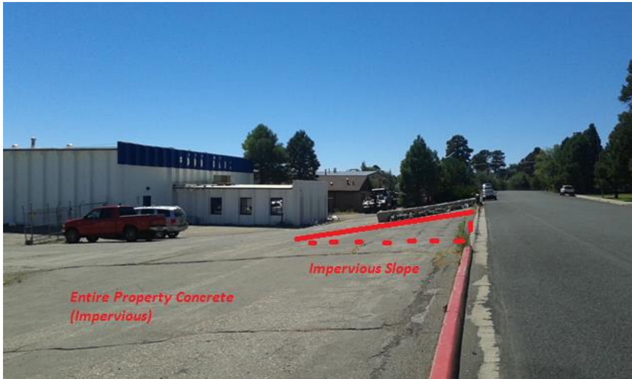
Figure 1.5 - Impervious Slopes & Surfaces
